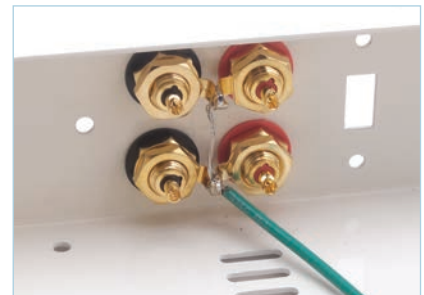
c. Run the long-stripped wire through both pairs of terminals, connecting the common grounds all together. Solder both pairs.
